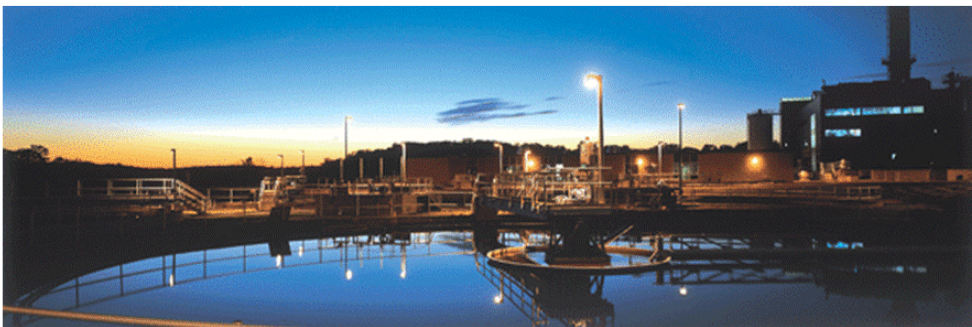
Prince William Service Authority – H.L. Mooney Water Reclamation Facility
